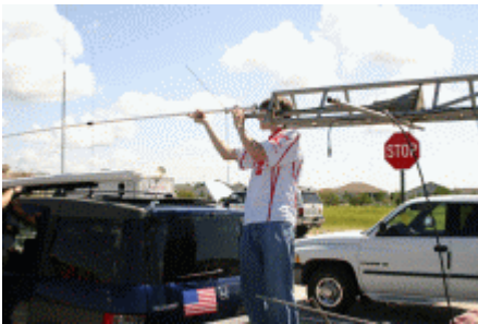
KG4JPL putting a dual band antenna on a crank up tower for a portable repeater.
